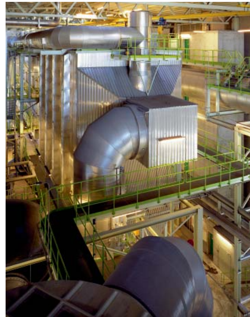
The combustion of waste releases considerable amounts of energy. A tonne of waste can replace around 350 kilograms of petroleum.
