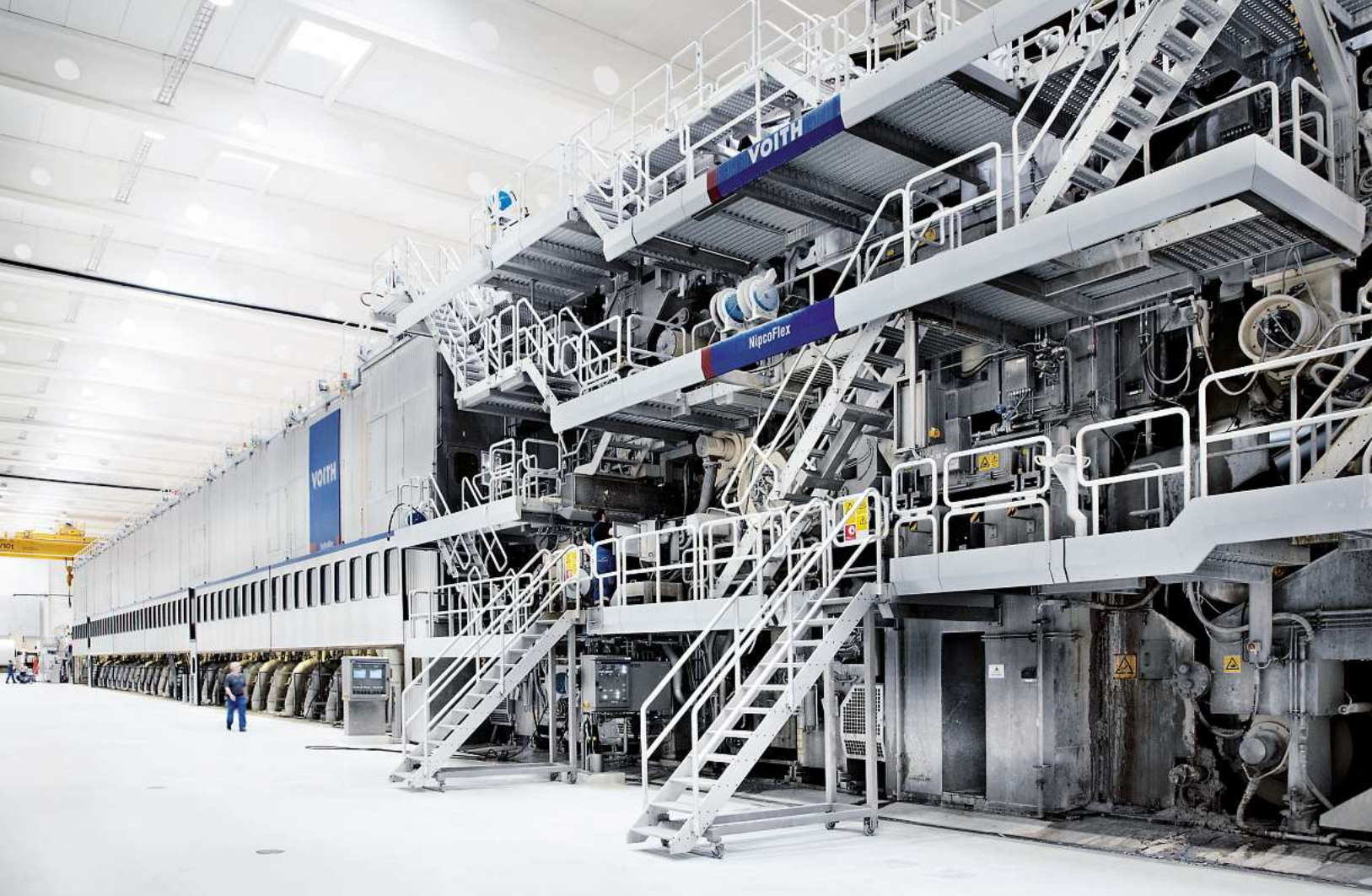
The 130-metre-long new paper machine for newsprint, called PM 7 is loud and unbelievably fast. Around 10,000 tonnes of steel was used to build the PM 7, about the same weight as the Eiffel Tower in Paris.
