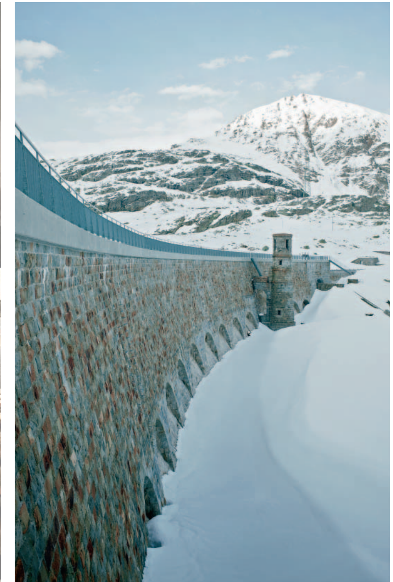
Dam heightening: the old south wall of the Lago Bianco reservoir.
