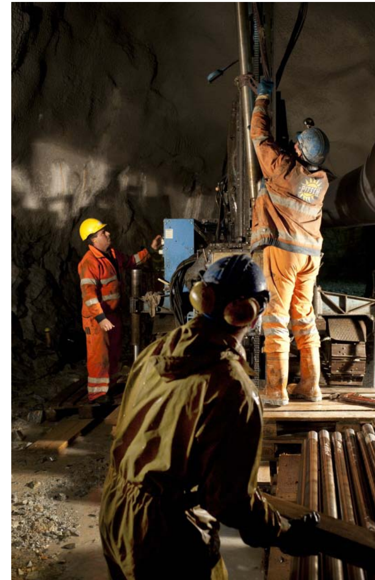
Exploration shafts: shifting in the stone can result in adjustments to the project.
