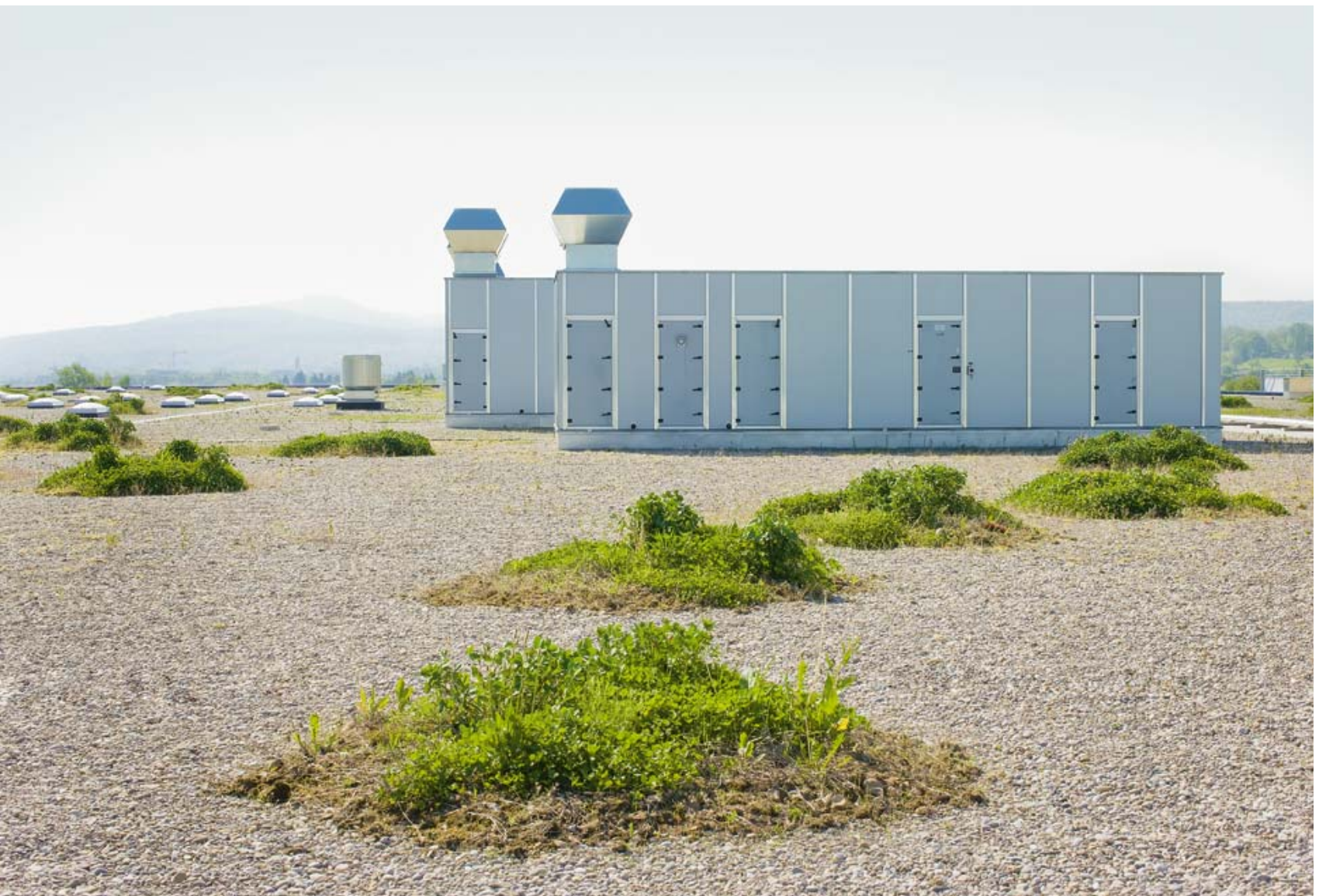
A 150-square-metre extendable solar system on the roof of the building in Spreitenbach ensures efficient use of energy. The roof has been planted with greenery to compensate for the green area that was covered over. Green “islands” serve as habitat for micro-organisms.
