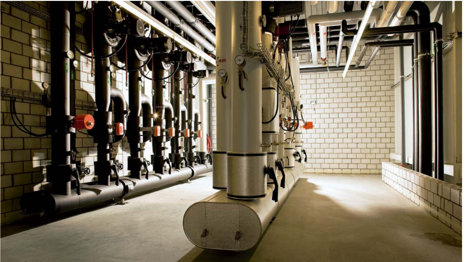
At the top, the building's heat and cold distribution system. The light system distributes the cold; the dark one the heat. In the photo on the right, the two furnaces powered by wood pellets – the largest of their kind ever to be constructed to date.
